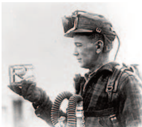
Left: Mining foreman R. Thornburg shows a small cage with a canary used for testing carbon monoxide gas in 1928. Right: Resuscitation cage with an oxygen cylinder serving as a handle used to revive a canary for multiple uses in detecting carbon monoxide pockets within mines. [Wikipedia]
